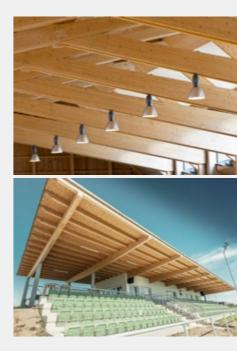
**GLULAM** is lighter than steel but has the same load bearing capacity. The natural power of the wood enables a slim dimensioning of the components.
